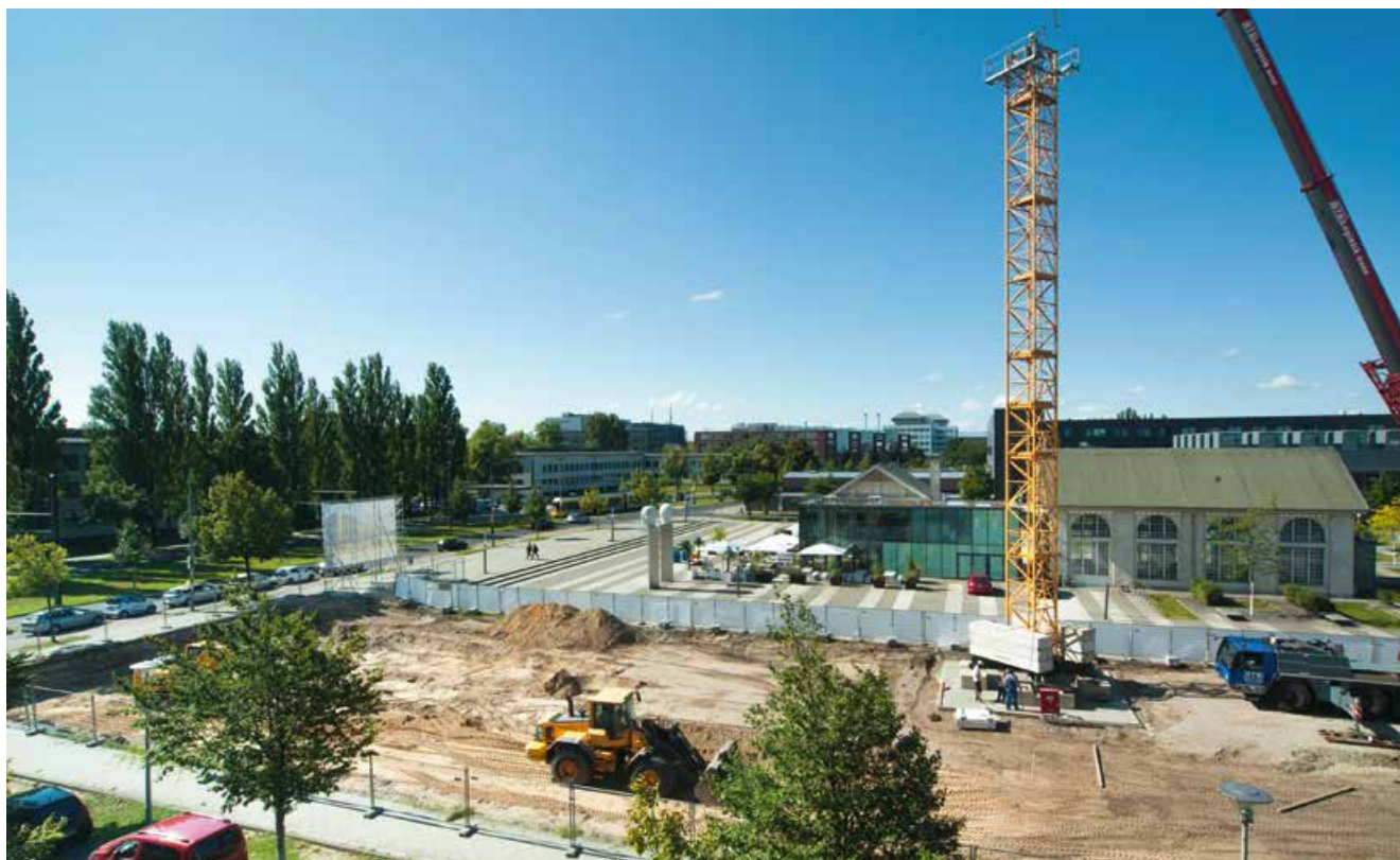
Baustelle EUROPA-CENTER am Forum Construction site EUROPA-CENTER am Forum
